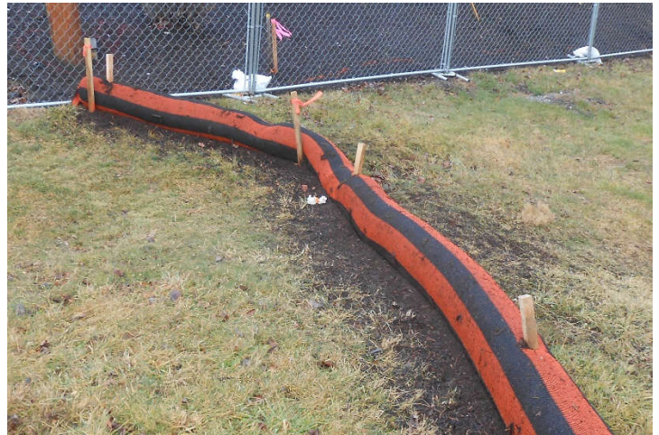
The silt sock above was not installed correctly. Improper ground contact, the lack of staking and mulch allows sediment to wash onto the adjacent sidewalk. It will cost time and money to reinstall. The silt sock below was installed correctly the first time. It will provide cost effective sediment control.
