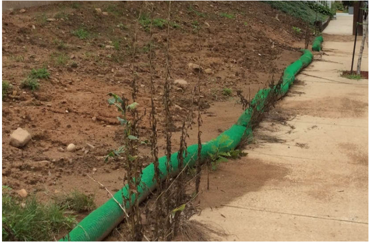
The silt sock above was not installed correctly. Improper ground contact, the lack of staking and mulch allows sediment to wash onto the adjacent sidewalk. It will cost time and money to reinstall. The silt sock below was installed correctly the first time. It will provide cost effective sediment control.
