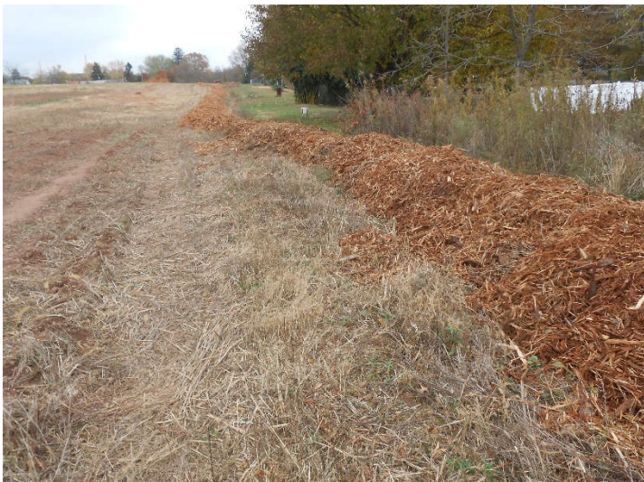
Mulch Berms, like the one shown above, are a great way to use on site materials as an erosion control practice. What was once a waste product from clearing and grubbing activities can now be used as an effective and cost saving way to prevent sediment from washing off a construction site.
